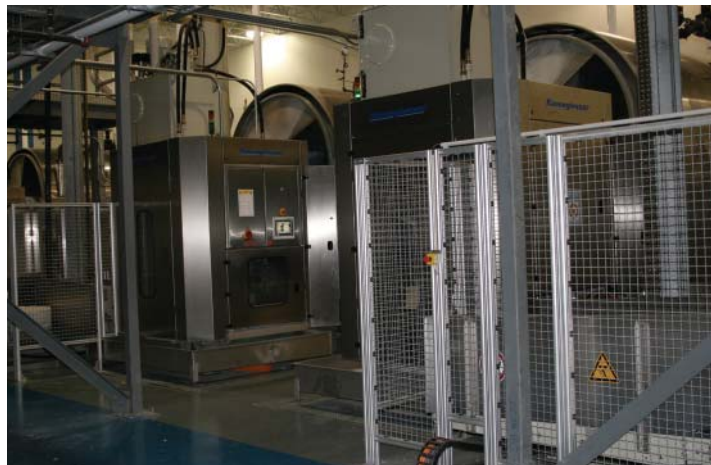
A view of three of the plant's four tunnel washers
