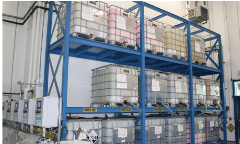
A view of the plant's chemical storage area, which is reinforced with heavy-duty shelving and metal-frame boxes to reduce the risk of spills in case of earthquakes
