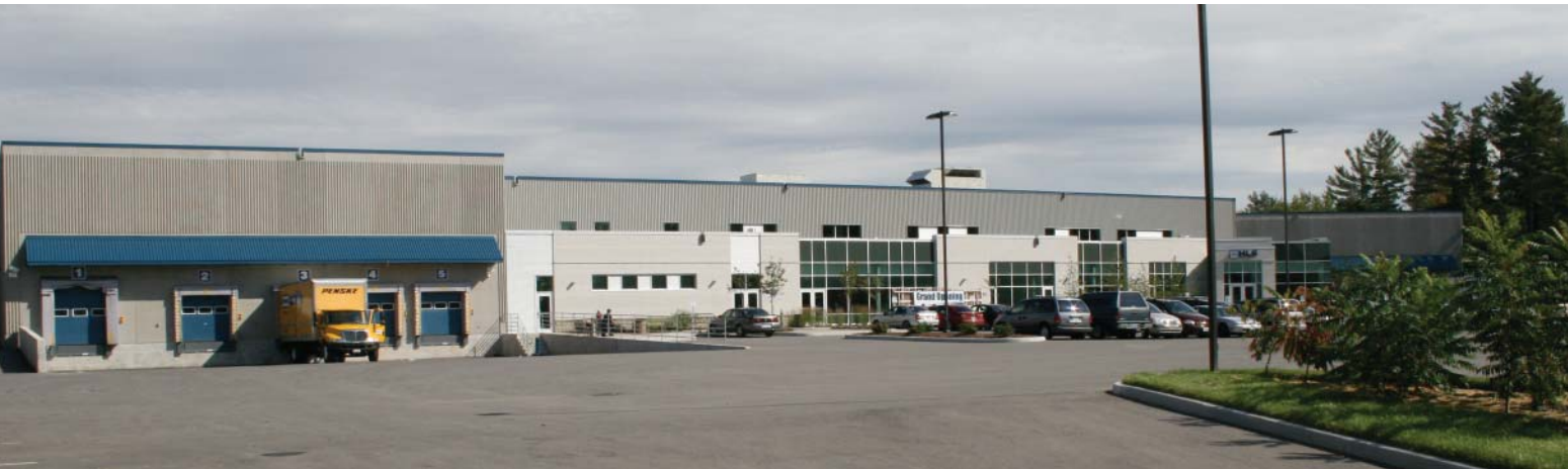
Here is a side view of the plant, including loading bays. HLS was constructed earlier this year on a 13-acre site. Company CEO Rocco Romeo and COO Pete Rainville worked with a team of architects and consultants to build a plant that would meet their short- and long-term needs amid growth in their healthcare and hospitality markets.
