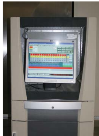
A computer monitor lets employees see where goods are in the tunnel washer.
